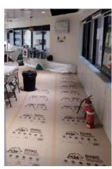
Temporary surface protection is designed to protect surfaces from superficial damage. Users should ensure that the substrate can take the weight of any equipment or materials being used regardless of protection being in place.
